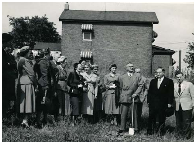
Breaking Ground at Regent Street Centre, 1955
